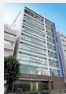
Akasaka 4-chome Building (Tokyu Agency Inc. Head Office Building)
