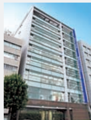
Akasaka 4-chome Building (Tokyu Agency Inc. Head Office Building)
