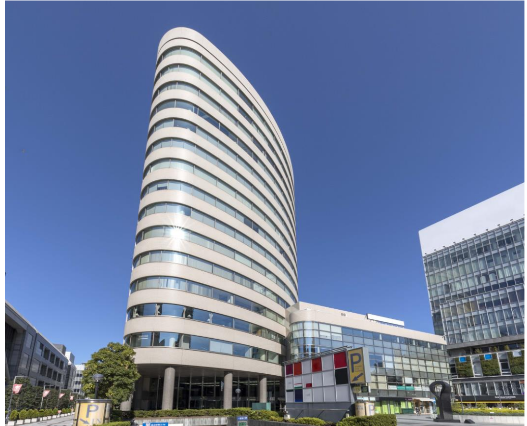
Aoyama Oval Building
