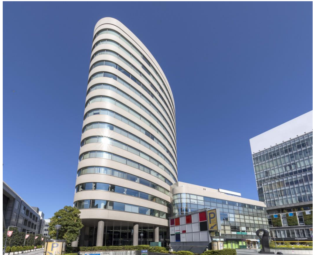
Aoyama Oval Building
