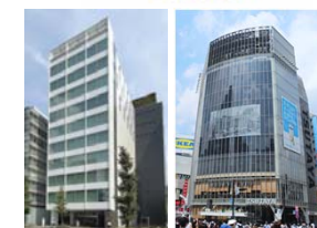
Tokyu Toranomon Building QFRONT
