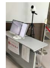
Installation of thermal cameras
