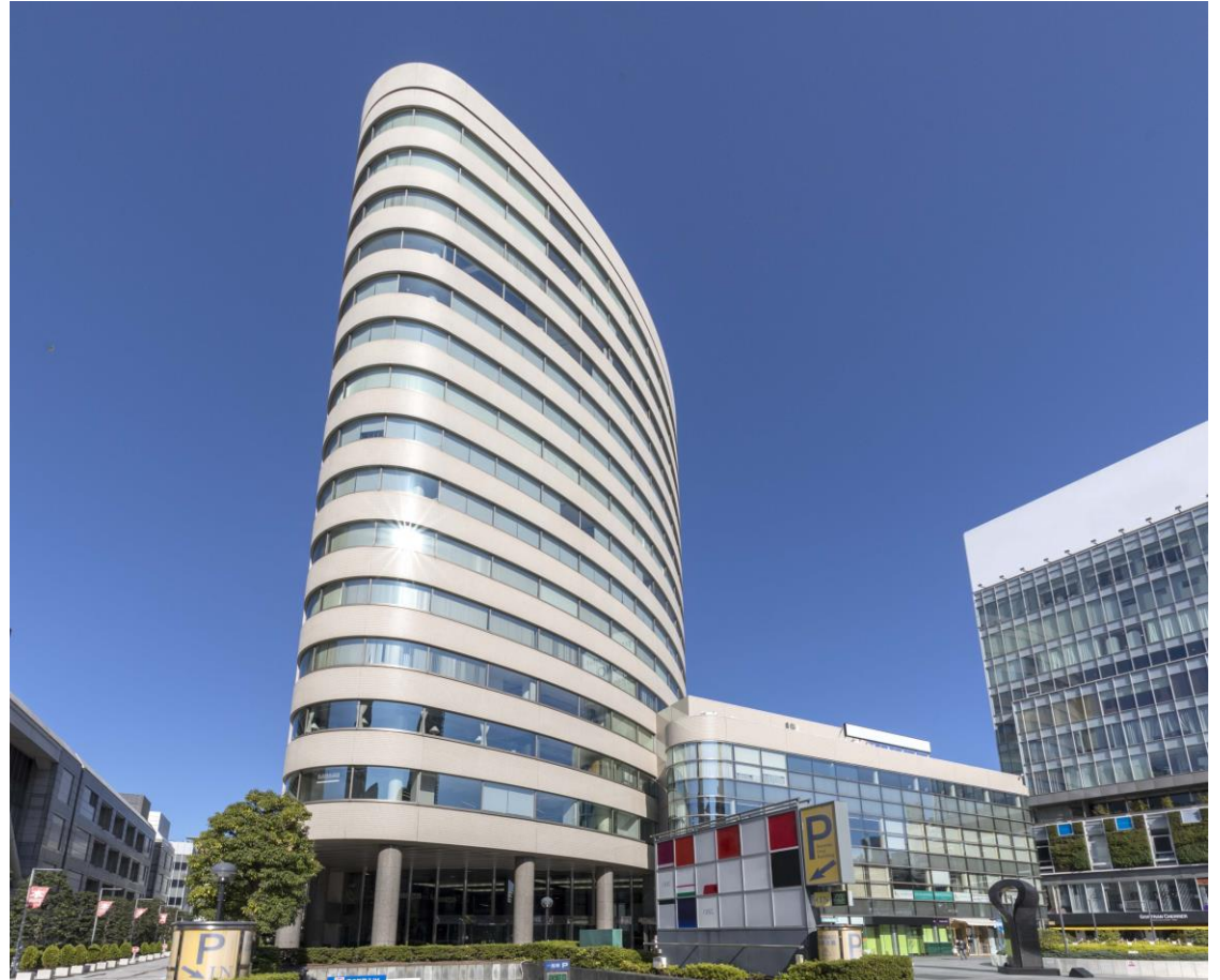
Aoyama Oval Building
