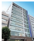
Overview of property
