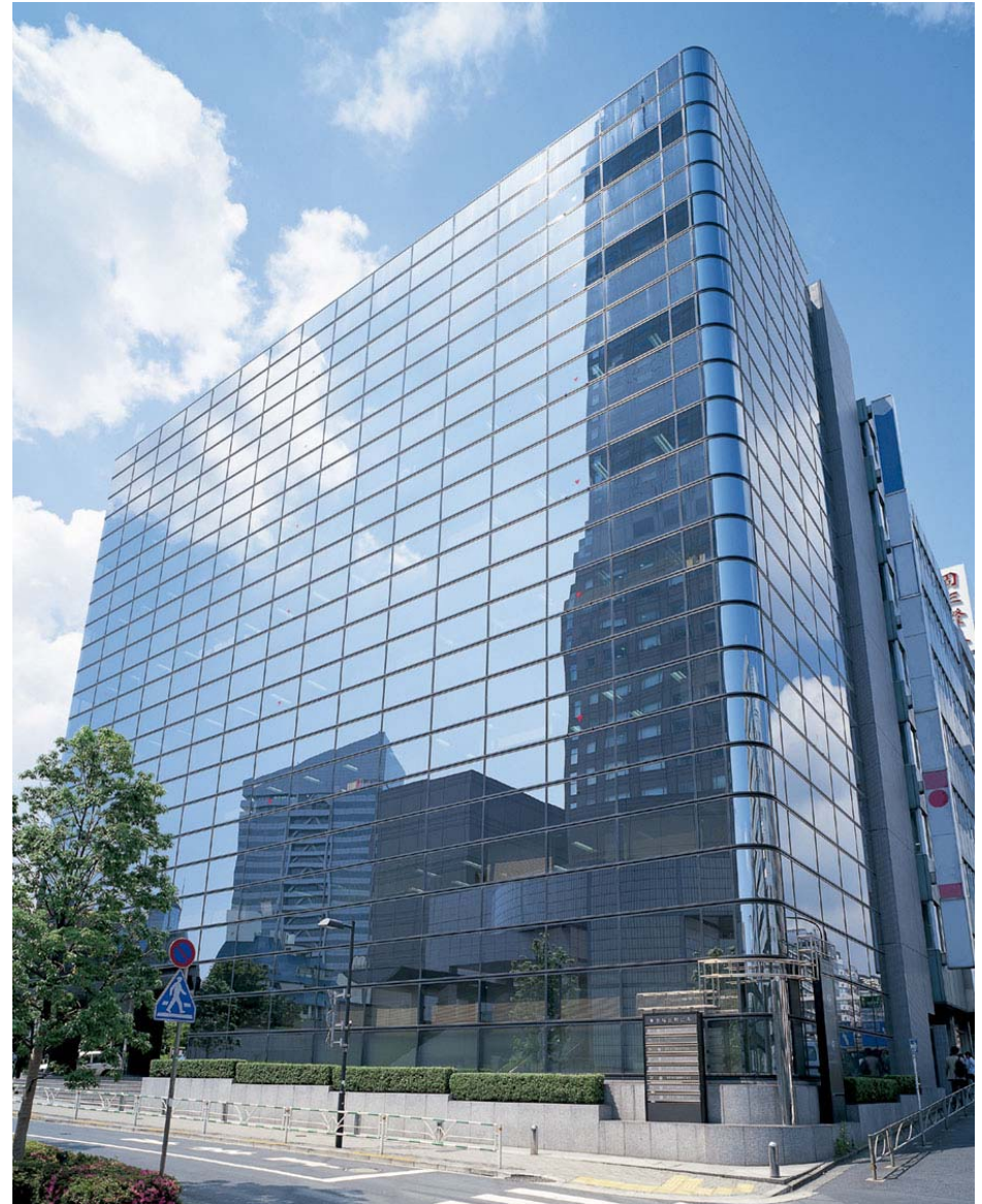
Tokyu Sakuragaoka-cho Building
