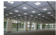
After construction work for switching to LED (Setagaya Business Square)
