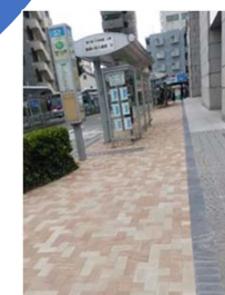
Laying of heat insulation interlocking block (Setagaya Business Square)
