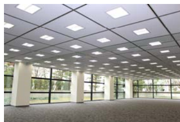
After construction work for switching to LED (Setagaya Business Square)
