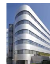
Tokyu Ikejiri-ohashi Building
