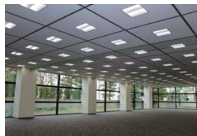
After construction work for switching to LED (Setagaya Business Square)
