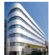
Tokyu Ikejiri-ohashi Building
