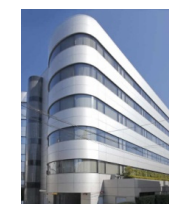
Tokyu Ikejiri-ohashi Building
