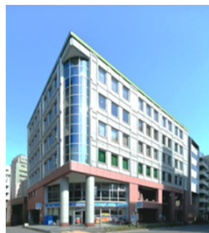
Overview of property
