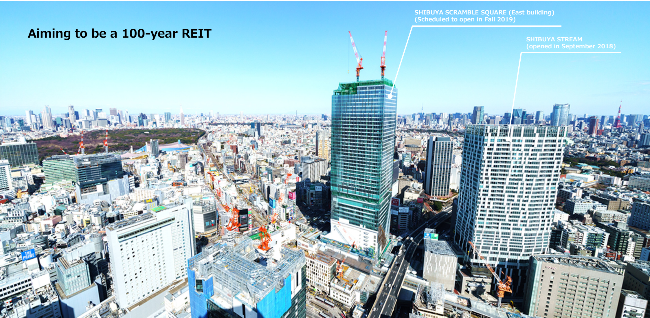
Status of Development surrounding Shibuya Station (photographed in February 2019)
