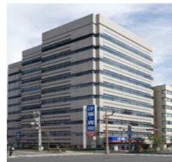
Overview of property
