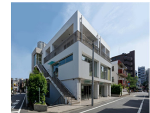
Overview of property
