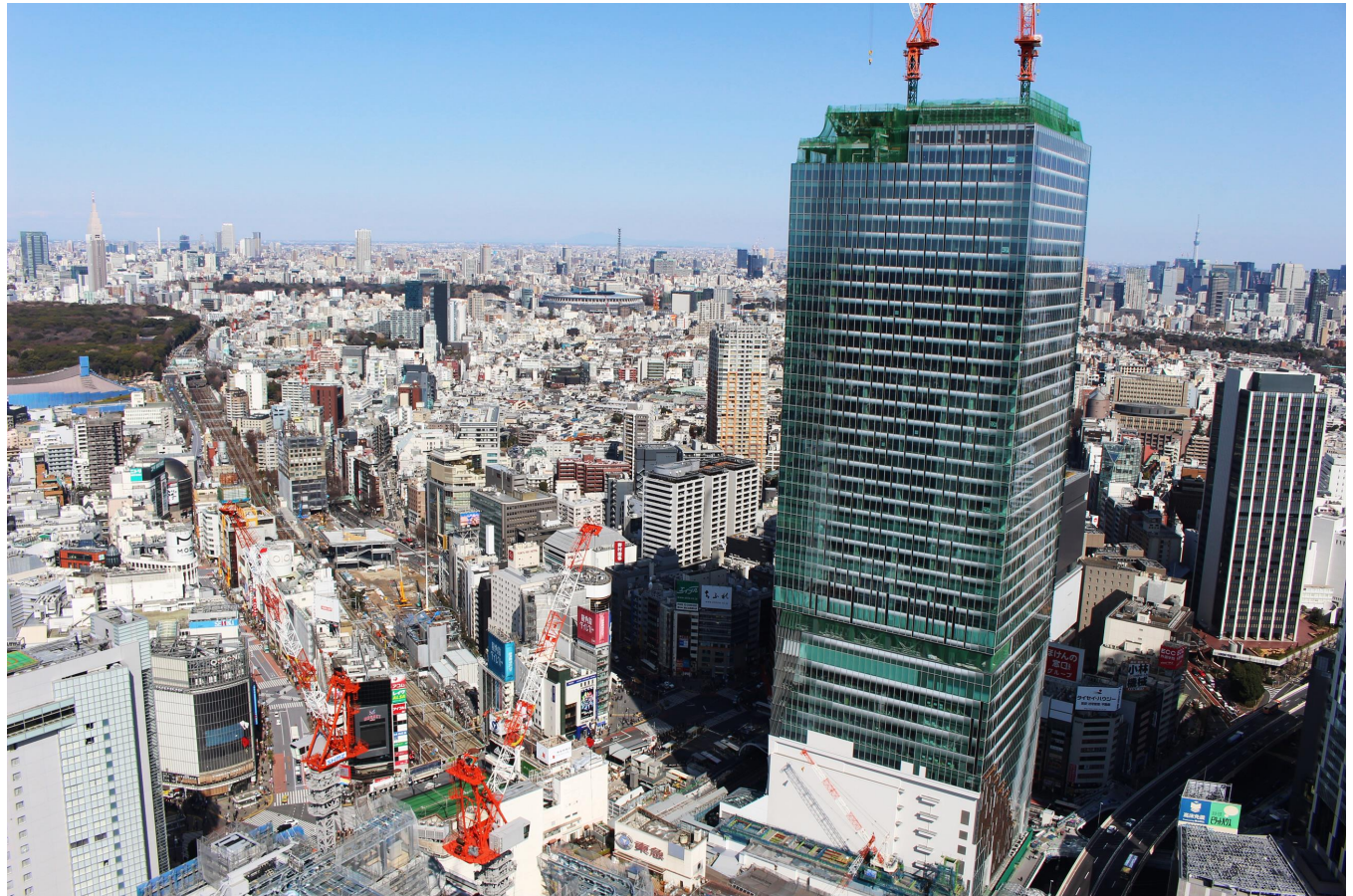
SHIBUYA SCRAMBLE SQUARE under construction
