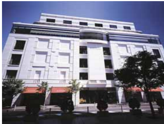
Yokohama Yamashita-cho Bldg. (Barneys New York Yokohama)
