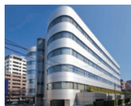
Tokyu Ikejiri-ohashi Building ★★
