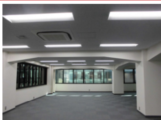
Interior after work to switch to LED and renewal of air-conditioning equipment (TOKYU REIT Hatchobori Building)
