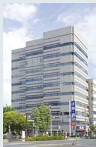
Kiba Eitai Building
