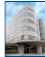
Tokyu Ikejiri-ohashi Building
