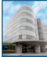
Tokyu Ikejiri-ohashi Building
