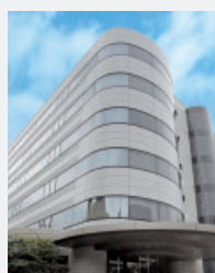
Tokyu Ikejiri-ohashi Building
