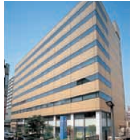
TOKYU REIT Kamata Building
