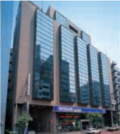
Tokyo Nissan Taito Building
