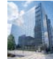
Tokyu Sakuragaoka-cho Building
