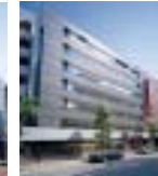
TOKYU REIT Akasaka Hinoki-cho Building
