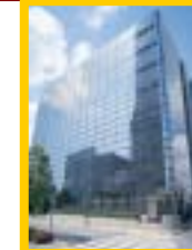
Tokyu Sakuragaoka-cho Building
