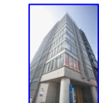
TOKYU REIT Shinjuku Building
